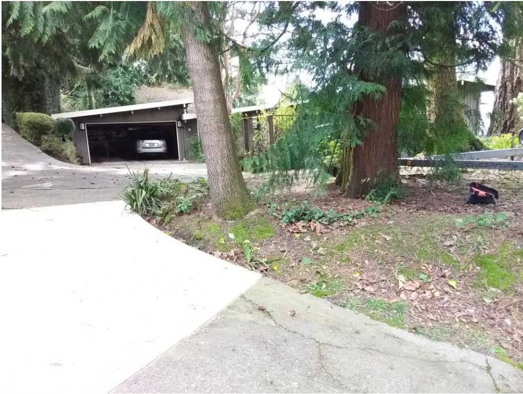
Figure 49. Area of new concrete east of the #30 and #31.
