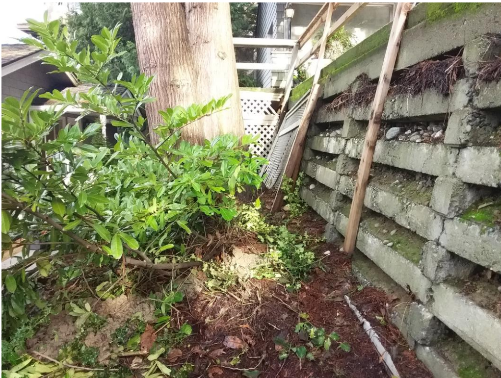
Figure 2. Looking north down the line of the retaining wall system that supports the lower parking area and the garage.
