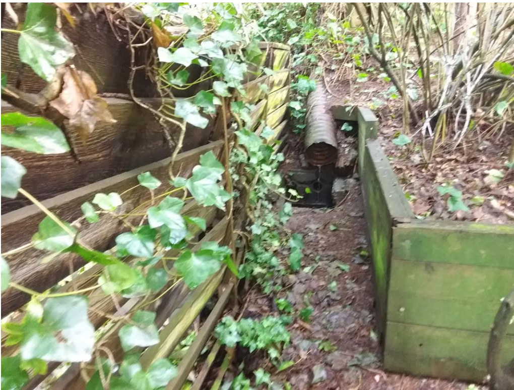
Figure 19. Looking east at the drainage system
